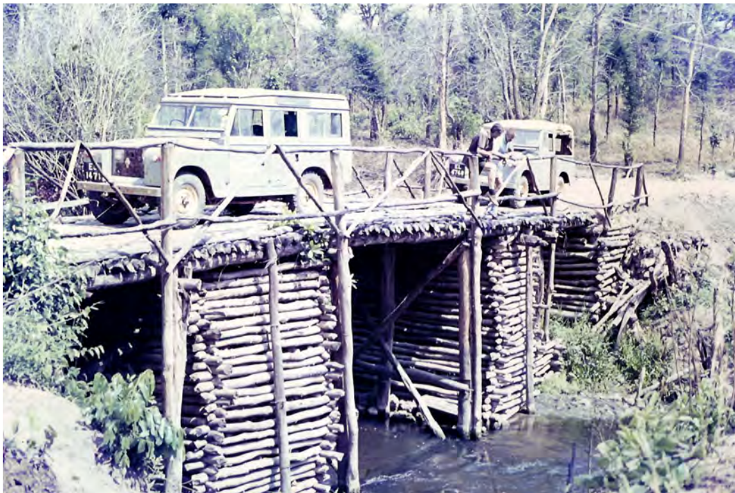
Bridge construction in a feeder road, Mpungu region 1970's, later the bridge was constructed with concrete pillars.
